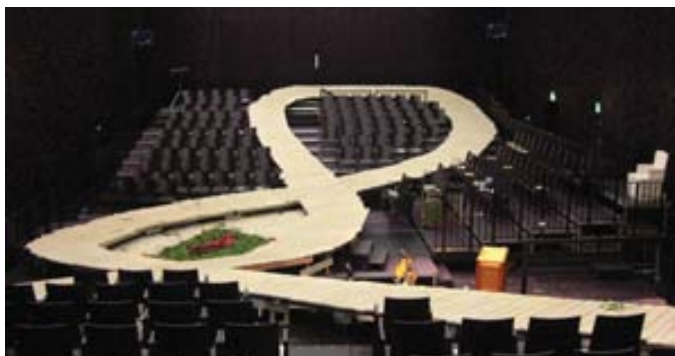
Each 2m x 1m section of floor has its own scissor lift, making the space hugely flexible
