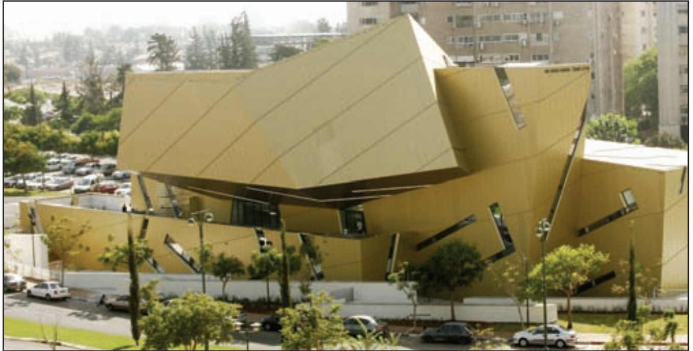
The Wohl Centre – The book-shaped auditorium is supported by two almost-rectangular boxes. (photo: Yoni Reif)
