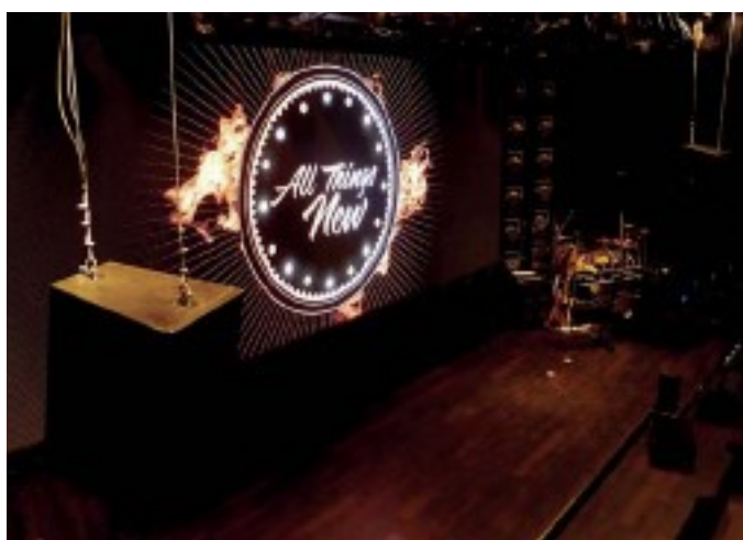
A suspended L-R Meyer Sound CQ1 system is supplemented by two HP700 subwoofers below the stage
